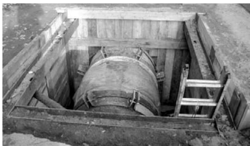
Water main from 1929
